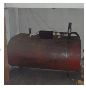
Figure 49: Above Ground Storage Tank (Source: T&M)
