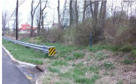
Figure 26: Stormwater Runoff Source - Inlet
